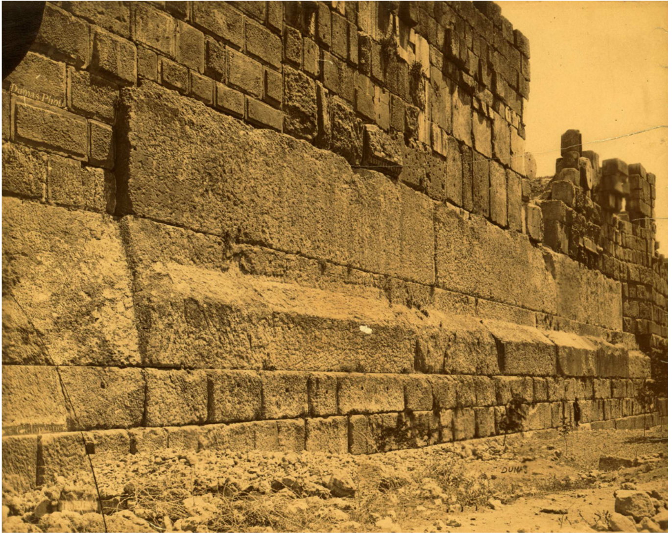
Photo. 8. Three “trilithon” blocks and a course of large plinth blocks below them on the west side of the Temple of Jupiter. The trilithon blocks are estimated to weigh 800 tons, and the plinth blocks 350 tons. Since the three courses of stone blocks of the fortress wall rest against the ends of the trilithon blocks on either side, the regular bonding pattern is disrupted in these places, thereby increasing the chances of wall collapse on both sides during an earthquake. In addition, in two other locations, the stone blocks of the wall above the trilithon blocks (north and south) are laid with gross violation of the bonding rule. How could the indicated bonding violations occur if the fortress walls were erected much later than the temple podium? Photo by T. R. Dumas, 1860, loc.gov.
