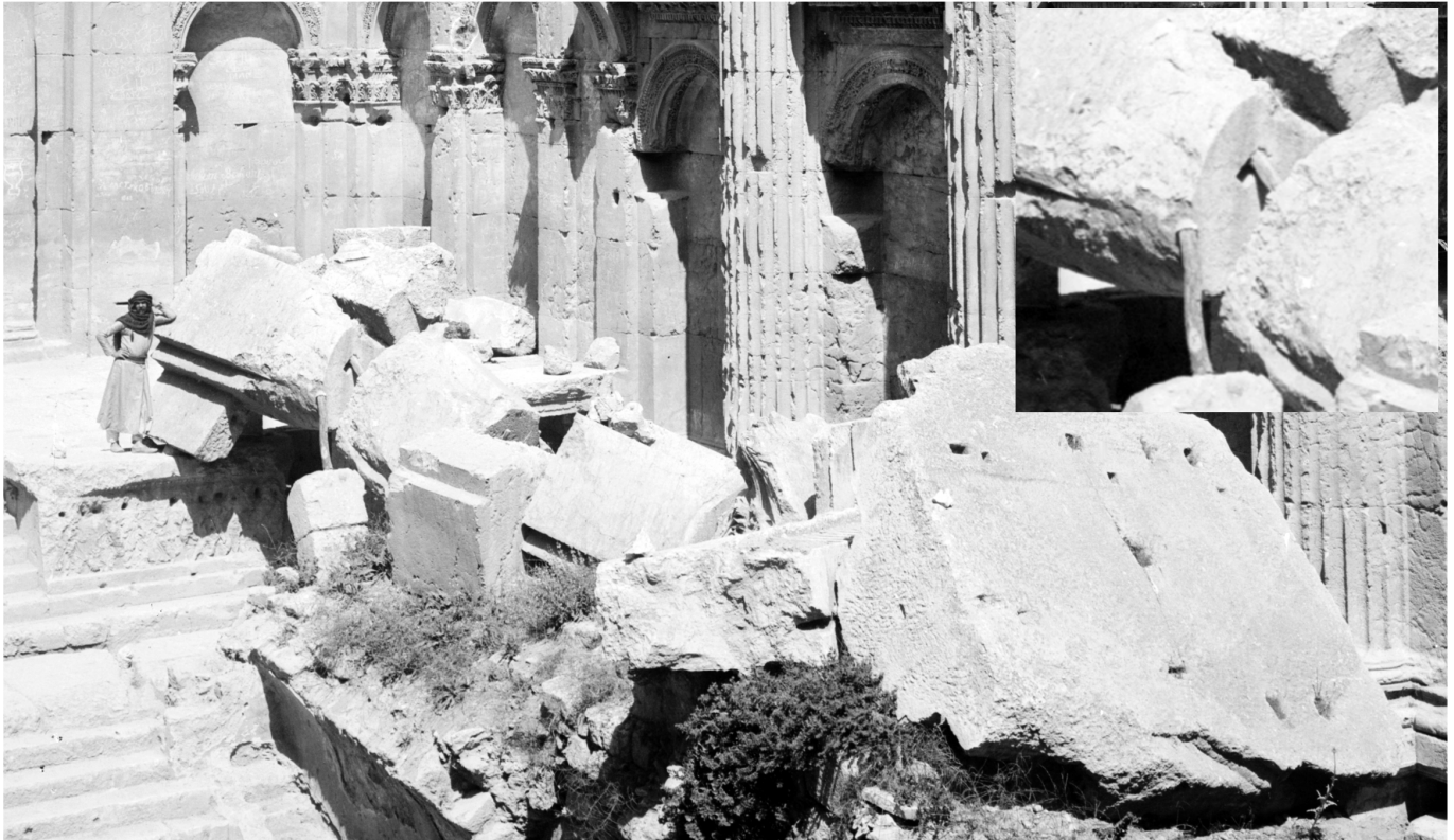
Photo. 20. A collapsed construction element in the Temple of Bacchus with “mysterious” rectangular and square holes from which protrude long metal reinforcing bars of large cross-sections (see the end face of the farthest block from us). Judging by the volumes of concrete casting and the type of reinforcement used, the “ancient Roman” temple was erected in the era of industrial production of iron and large-scale products of it. Photo from site of the Library of Congress, 1898, loc.gov.
